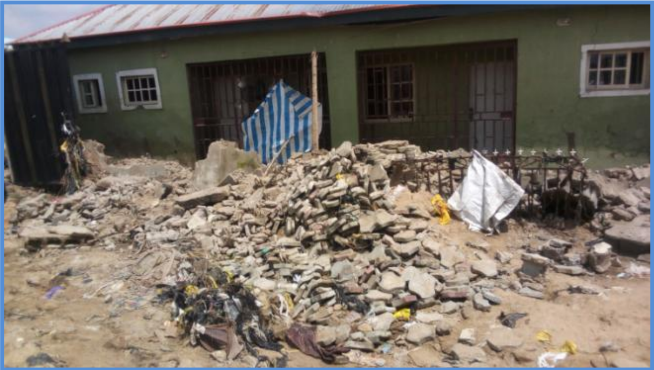
PLATE 13: INTERLOCKING TILES REMOVED BY FLOOD
