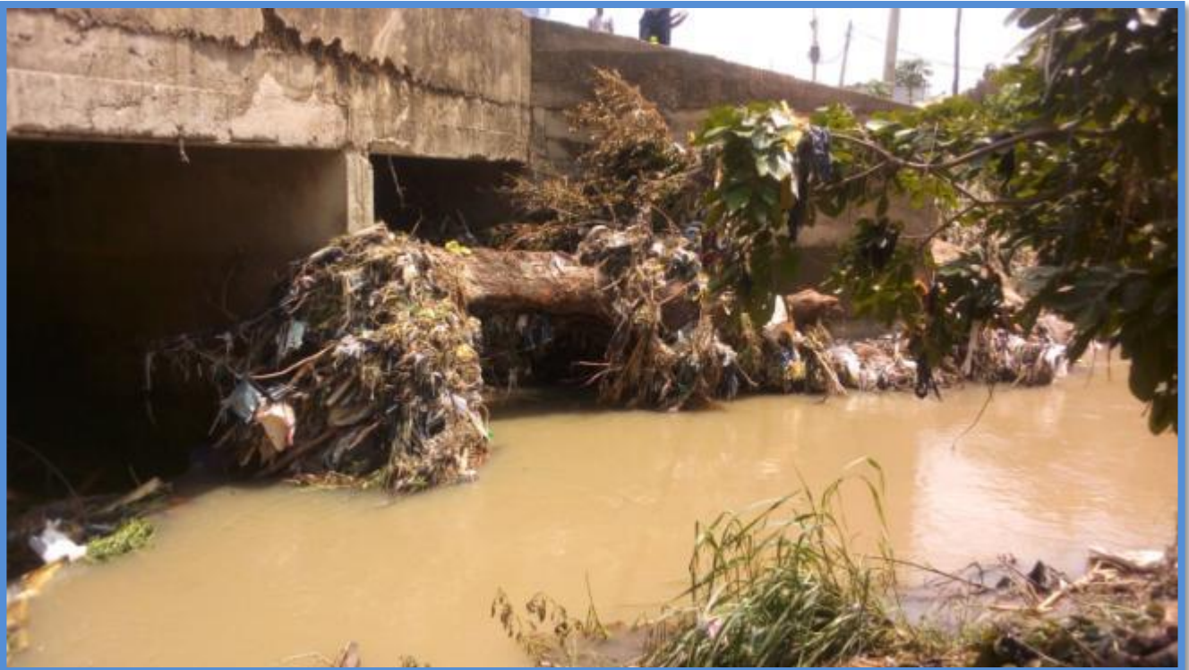
PLATE 8: DRAINAGE BLOCKAGE AT YARO BRIDGE
